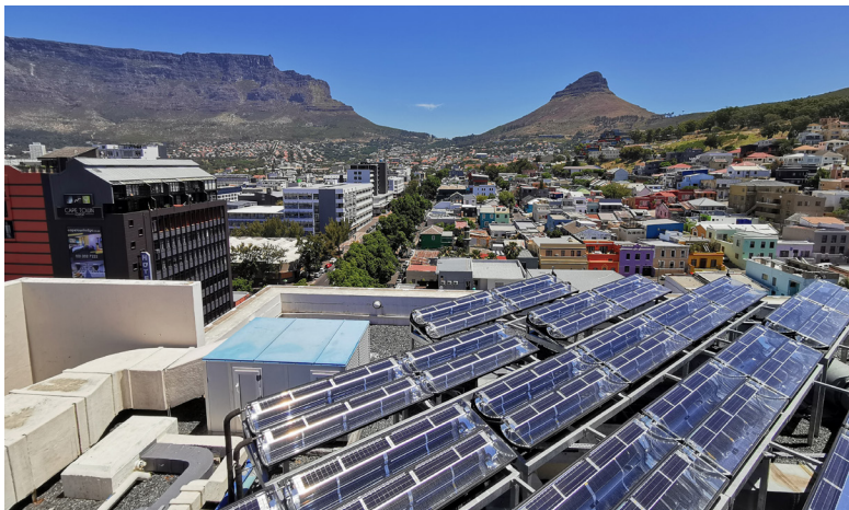
The hybrid Photovoltaic and Thermal system at the Hilton Cape Town City Centre produces clean energy for the hotel.
